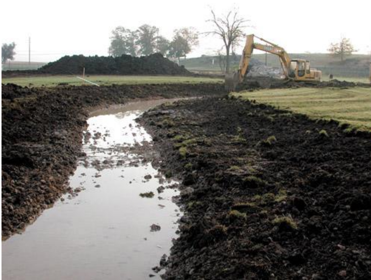
Example of widening the channel
