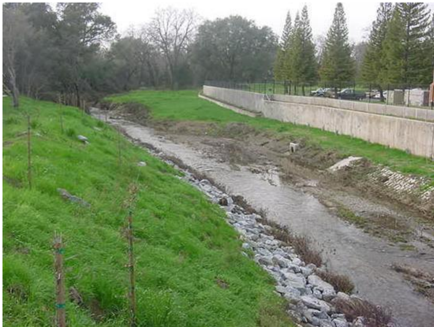
Example of the construction of flood walls
