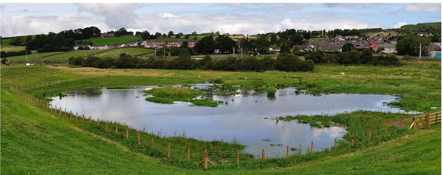
Example of a typical flood storage reservoir
